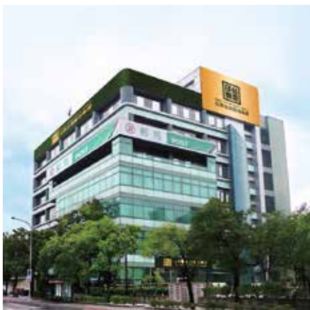
Nangang Post Office
