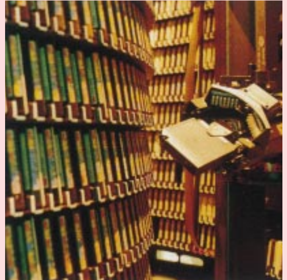
自動化磁帶管內機 An internal view of Automated Tape Library
